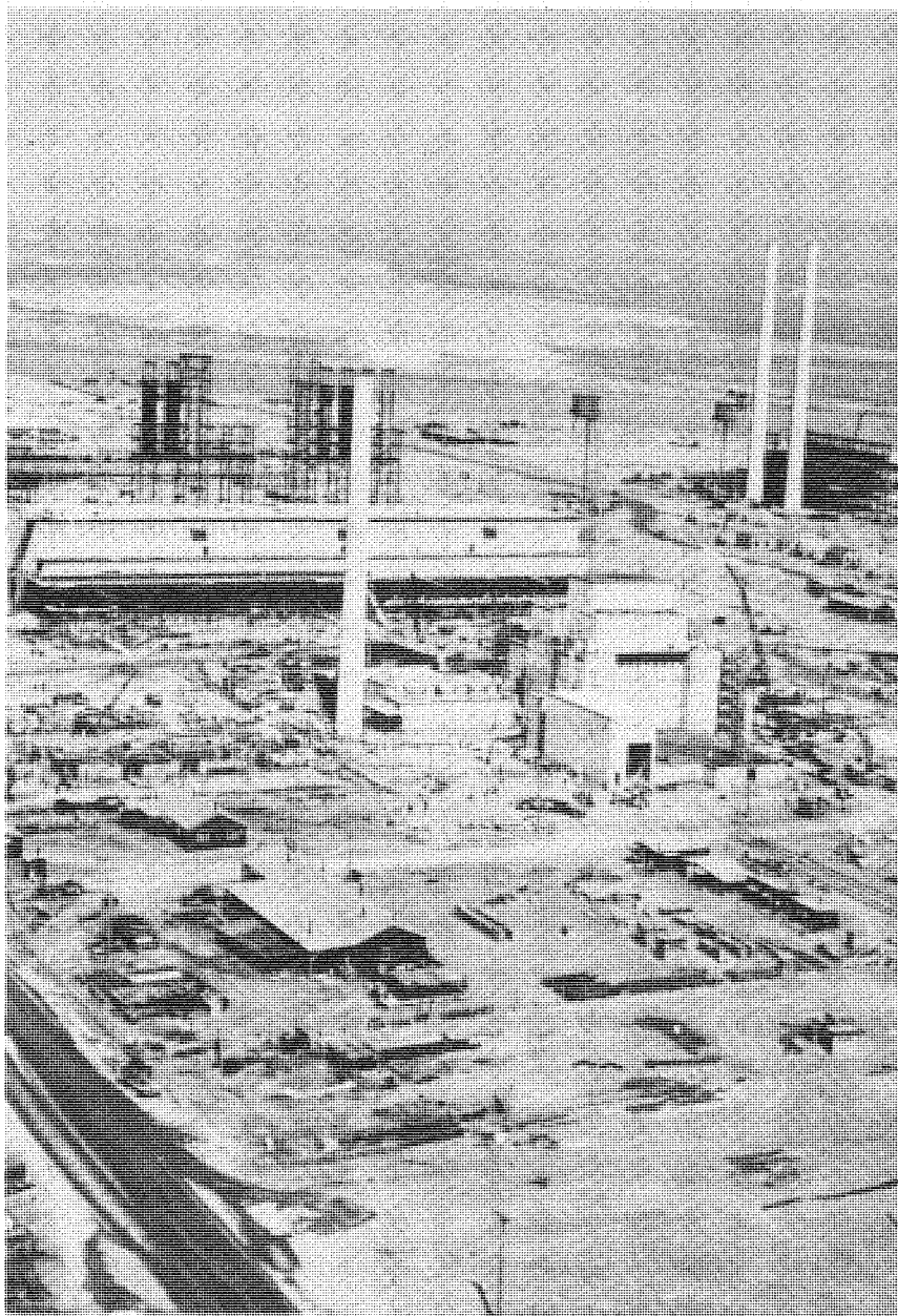
HANFORD D PILE AND SUPPORTING FACILITIES, JUNE 20, 1944 / The pile building, which towered 120 feet above the desert, is the concrete structure in the center. Behind it lies the water-treatment facilities. The Columbia River and the Wahuake Slope are in the background.
