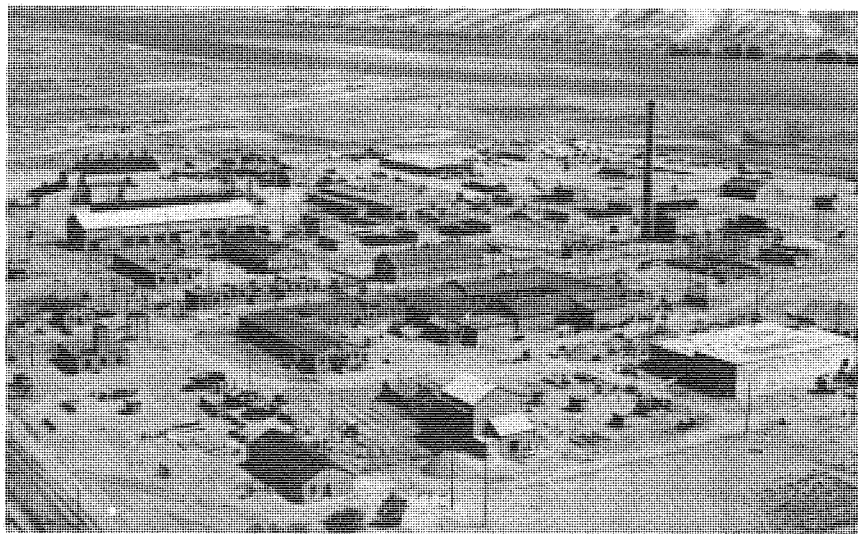
300 AREA AT HANFORD / Here du Pont manufactured uranium slugs and tested materials for the production piles. Slugs were fabricated in the one-story masonry building in the center background. Materials were tested in a 30-watt pile in the large vented building at the upper left.
